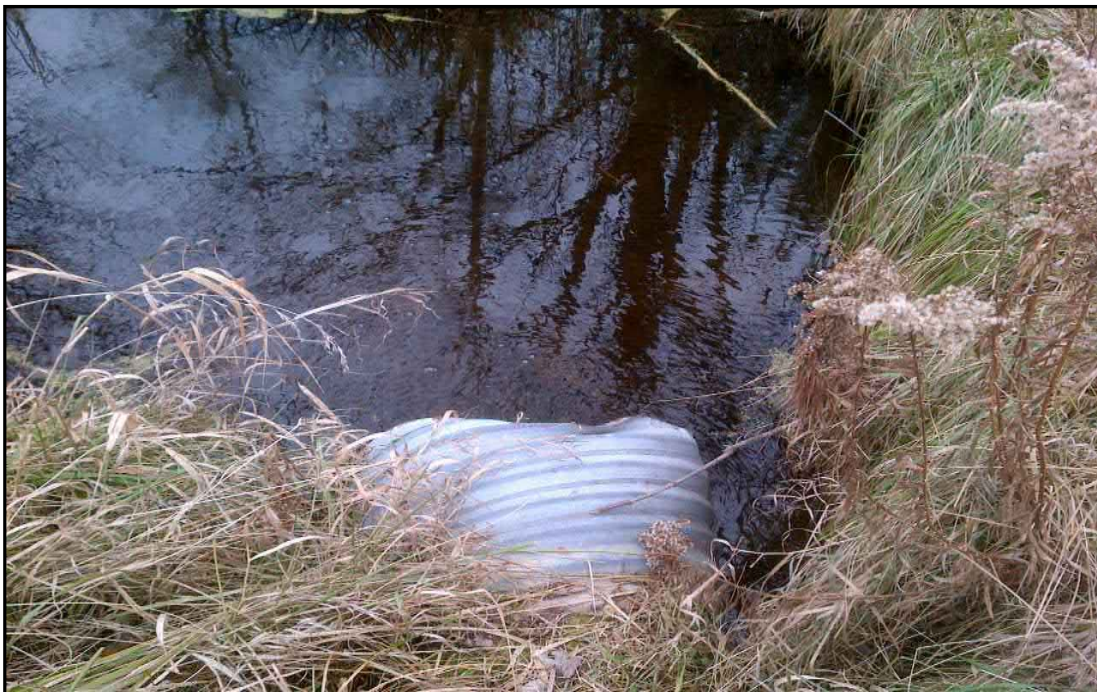
Photo 3 Cowan Drain at Oxford Road 3 Crossing taken on December 6, 2013
