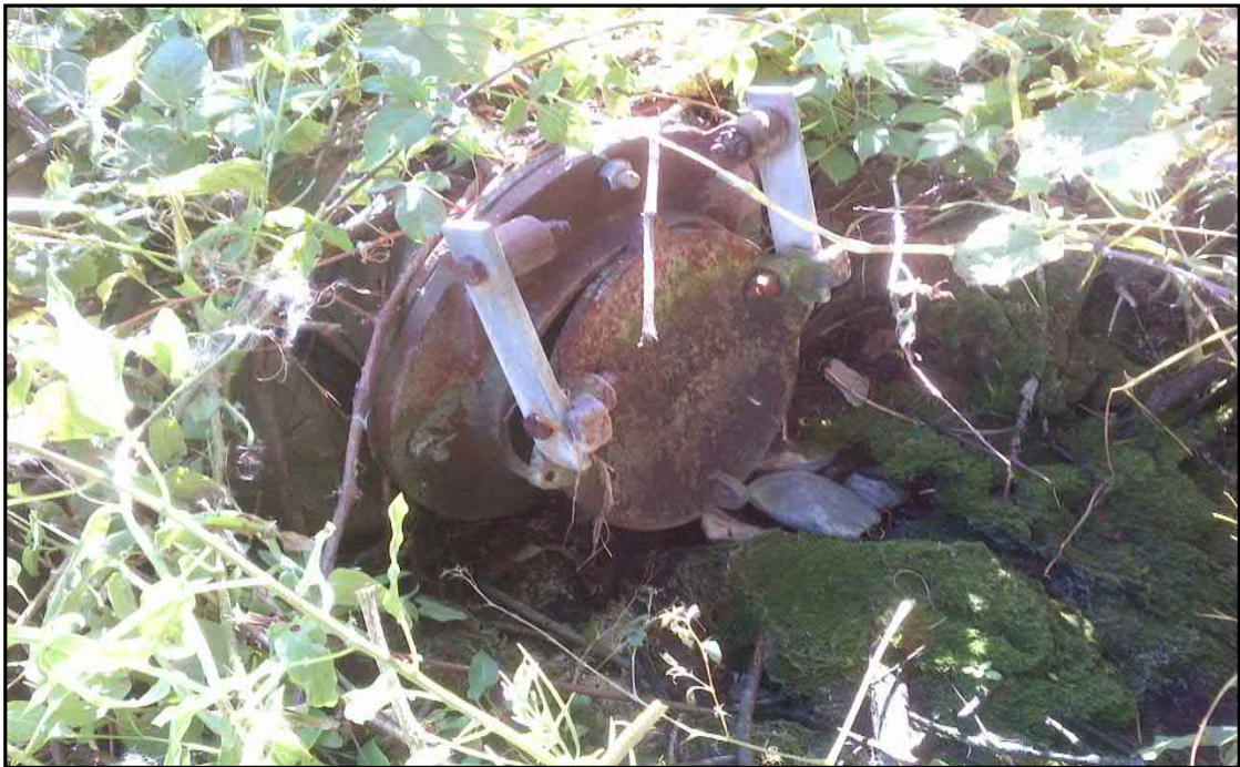
Photo 1 Photo of Outfall Pipe taken on September 25, 2013
